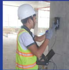
Non-Destructive Testing (NDT)
