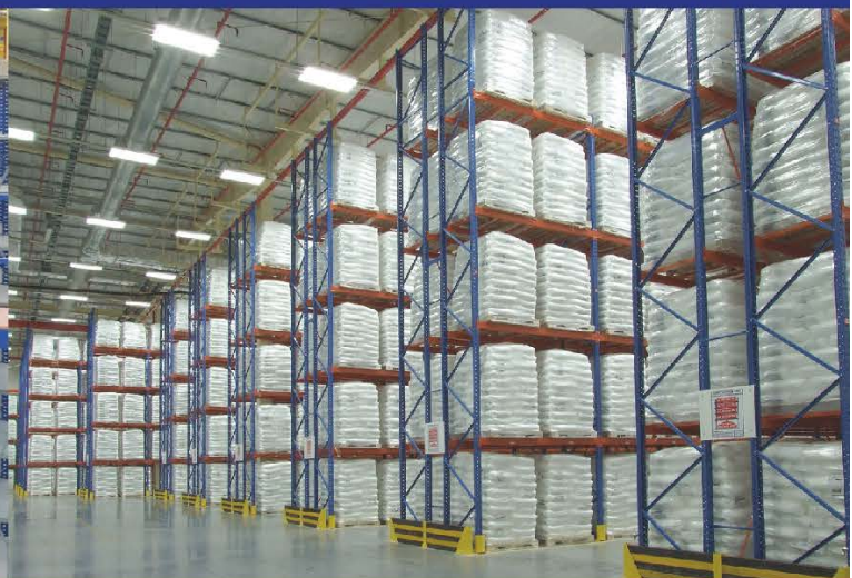
▶ Storage Racking Systems
